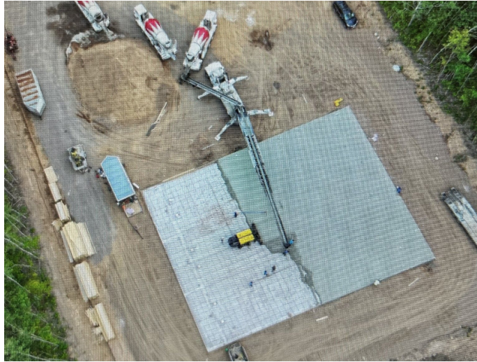
Slab pour, from above.
