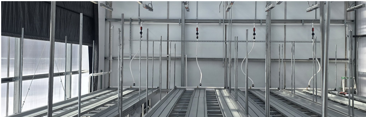
Greenhouse interior: rolling benches, irrigation, and blackout curtain.
