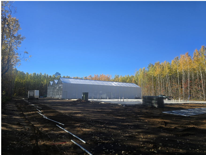
Greenhouse structure going up.
