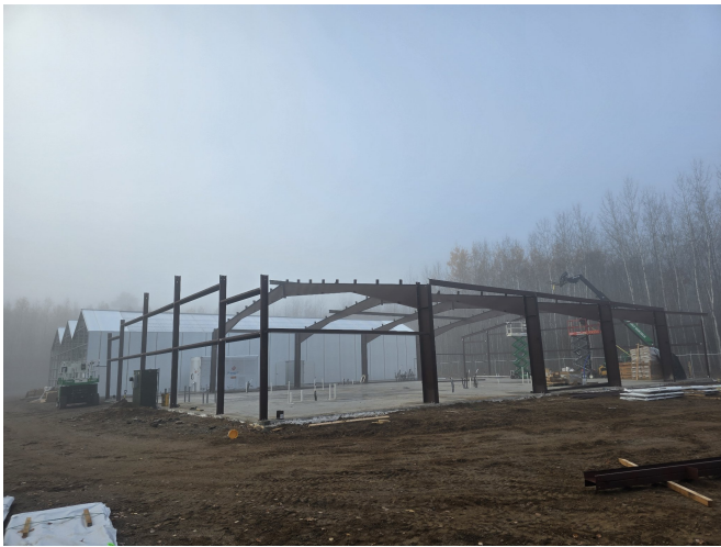
Steel frame rising.
