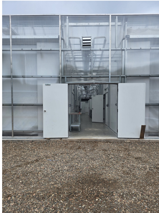
Greenhouse entrance and interior corridor.
